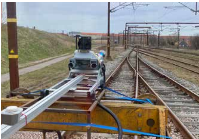
The mobile mapping system was mounted on the front of a rail maintenance lorry. LE34's tests determined to optimal speed for this mapping project, a function of survey control target spacing, and desired point density, was 45 to 50km per hour.
